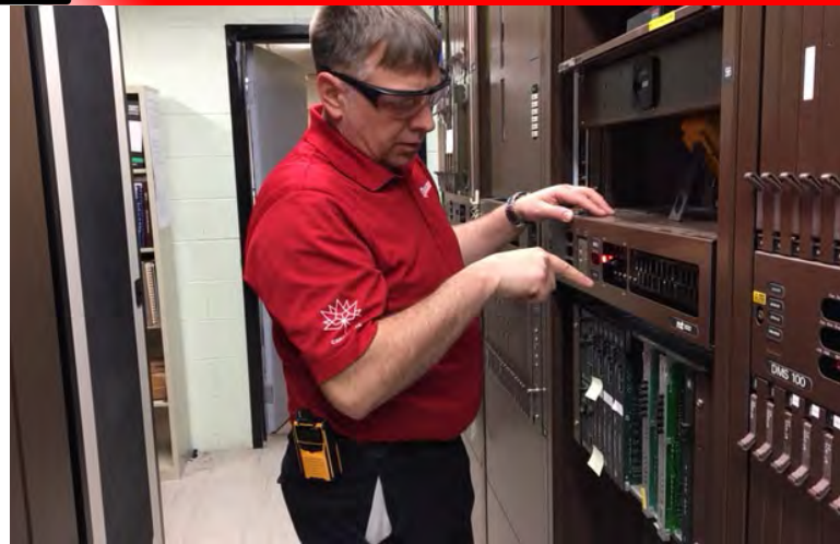
Barry Stone working on the removal of the old DMS 100 System.
